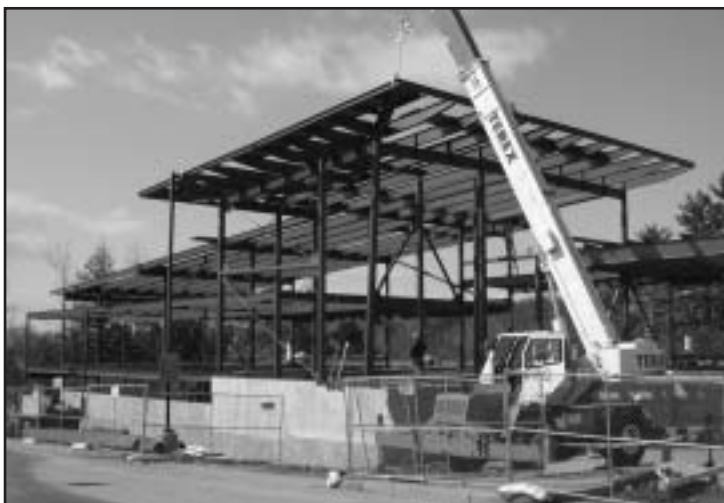
Construction of the new entrance to the John Mitchell Center.
